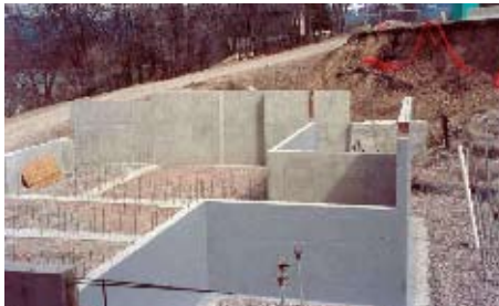
The first Solid Foundations pours went quickly and smoothly.
