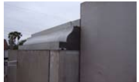
Forming the walls did not require a lot of special equipment.
