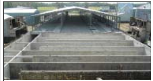
Over a mile of poured wall went into the final structure.
