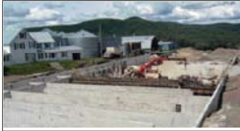
The dairy farm structure begins to take shape.
